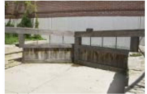
Reproduction of wooden canal lock doors
