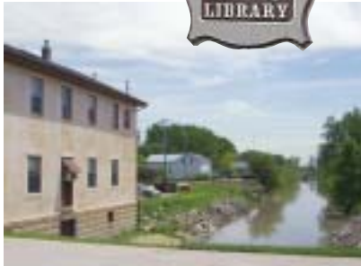
The Dutch Mill once received deliveries from canal barges directly through a side door.
