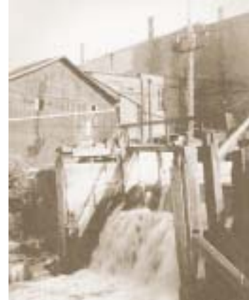
Original Lock 23 North
