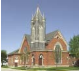
New Bremen has many restored canal-era brick structures in its historic downtown.
