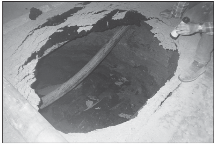
Subsidence pit, about 6 feet across and 8 to 10 feet deep, on I-70 resulting from roof collapse of a mine in March 1995. Photo courtesy of Gannett Fleming, Inc.
